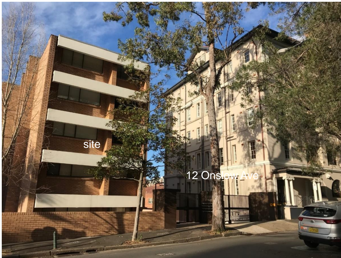
northern elevation of 12 Onslow Avenue
