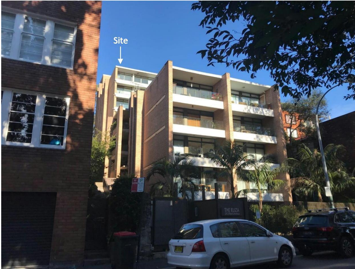
view of site from Billyard Avenue
